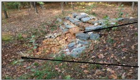
Materials can include a mix of granite or iron boulder to create the step-pools
