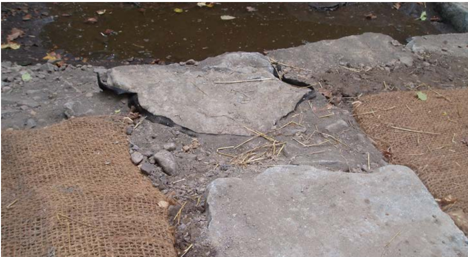
Figure 5. Vane rocks should fit snugly together and be chinked with smaller rock with a wide range of sizes. (Design by Wetland Studies and Solutions, Inc.)
