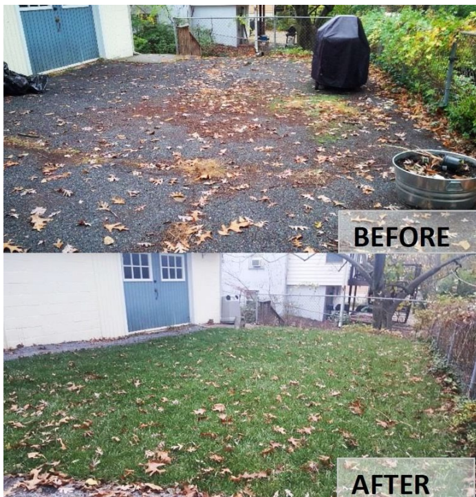
Figure 7. Pavement removal project before and after in the RainScapes Rebate Program.
