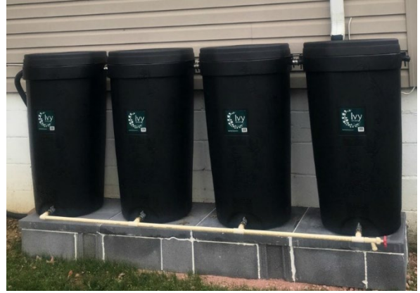
Figure 3. Four 50-gallon rain barrels connected together and installed at a residential property.
