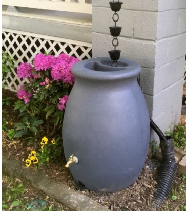
Figure 2. A 50-gallon rain barrel with a rain chain installed at a residential property.
