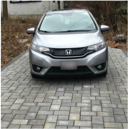
Figure 8. Pavement was removed and replaced with 360 square feet of interlocking permeable pavers at a residential property.
