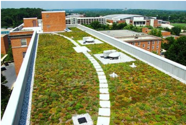
Figure 15. A green roof at the University of Maryland. This is an example of a green roof. This project was not funded through this program. (Photo credit: University of Maryland. https://sustainability.umd.edu/campus/water )
