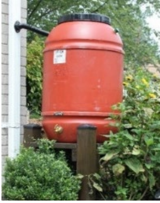
Figure 1. A 55-gallon rain barrel installed at a residential property.
