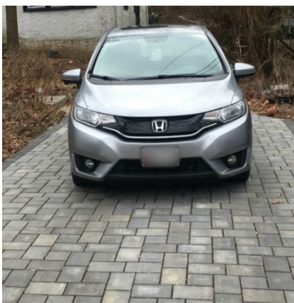
Figure 92. Pavement was removed and replaced with 360 square feet of interlocking permeable pavers at a residential property.
