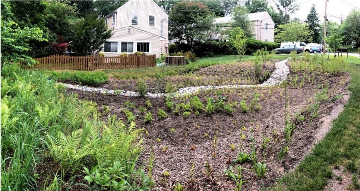
Several years ago, Greenbelt Homes, Inc. (GHI) received a grant to install a stormwater management system in the community. This system includes a stone diaphragm, stone swale, and rain garden that work together to intercept and capture runoff from the parking lot, sidewalk, and roofs of nearby homes. Since the installation, GHI has noticed significant improvements. The rain garden also offers a beautiful community space.
