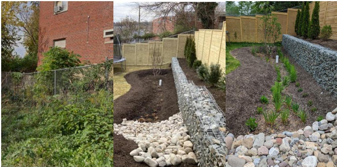
Rain gardens support water-tolerant native plants that soak up stormwater flowing from impervious surfaces. Stormwater management practices like rain gardens, trees, and removal of impervious pavement are successful in reducing stormwater runoff, and are even more successful when utilized together!
