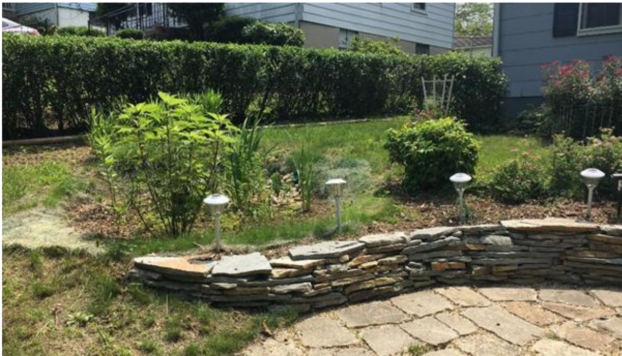
A rain garden, weep wall, and permeable pavement pictured at this residence will capture runoff flowing downhill and reduce flooding in their yard.
