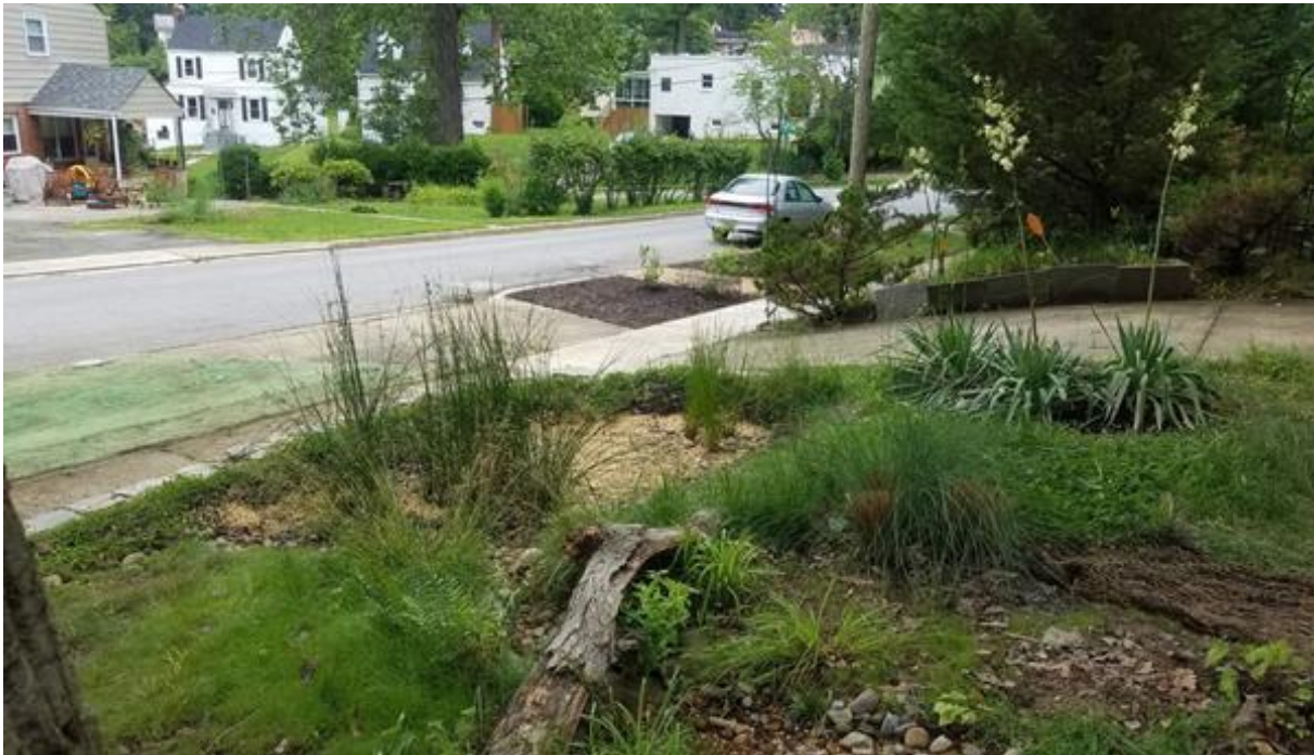
Stormwater runoff now flows into a dry stream that leads to a large rain garden.
