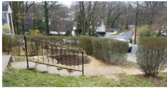
A rain garden installed at the adjacent corner of the uphill neighbor's yard slows down and captures runoff on site.
