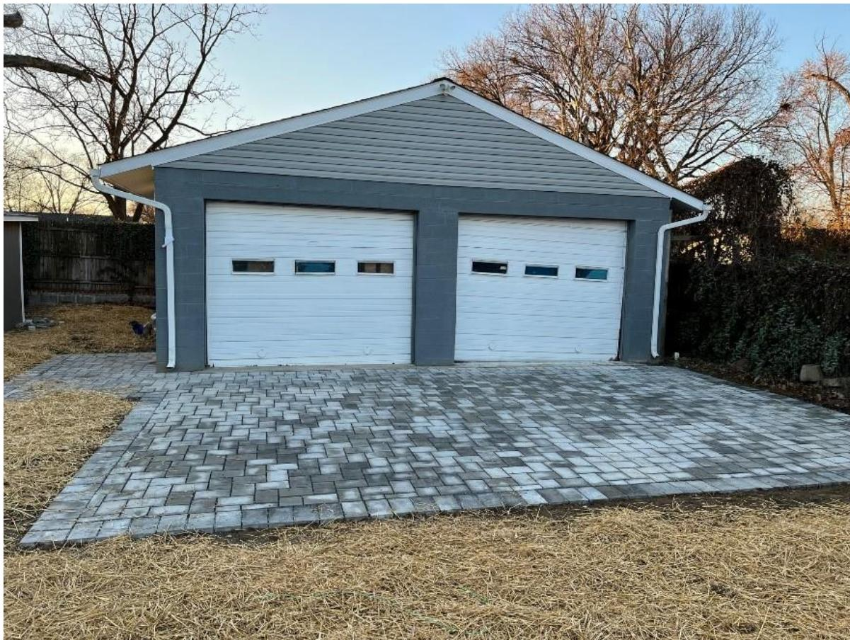
Unlike conventional asphalt or concrete, permeable pavement allows water to infiltrate and soak into the ground. A variety of permeable pavement materials are available, such as interlocking pavers, porous asphalt, pervious concrete, and manufactured grass pavers that include a storage system beneath the surface to capture stormwater runoff and allow it to soak into the ground beneath.
