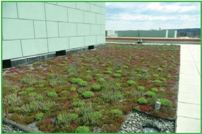
Green roofs can be extensive or intensive. Extensive green roofs require 2 to 6 inches of engineered soil medium and support a variety of low-growing, drought-tolerant plants.
