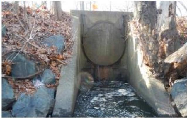
Lockridge Drive Tributary 48" RCP storm drain (SD) outfall with concrete wing walls (looking upstream)
