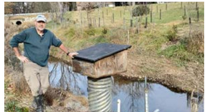
PLBR stormwater monitoring station
