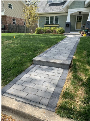
Figures 8 & 9. Permeable Pavers installed through the City of Rockville RainScapes Rebate Program.
