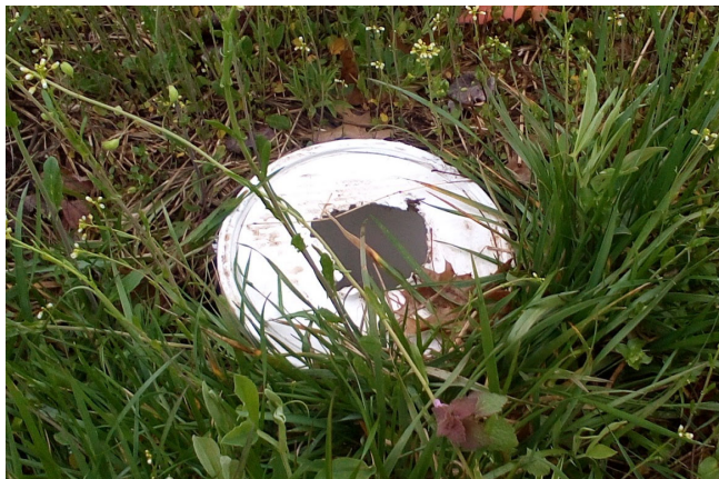
Figure 7. Photo showing evidence of tampering with cap on underdrain clean-out pipe at EC-BS2.
