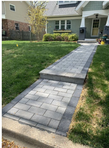
Figures 8 & 9. Permeable Pavers installed through the RainScapes Rebate Program.
