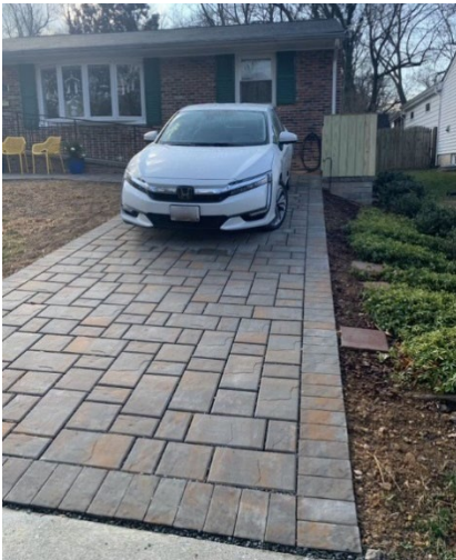
Figures 8 & 9. Permeable Pavers installed through the RainScapes Rebate Program.
