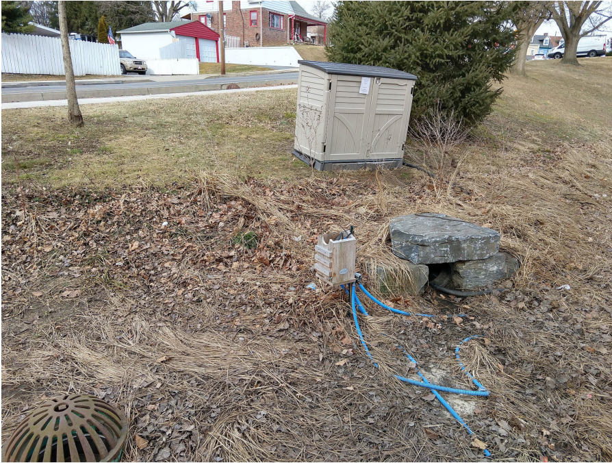
Field study w/ two basins w/ different salt loading in Lancaster, PA
