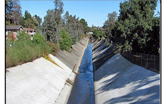
Concrete-lined sewer (channel)
