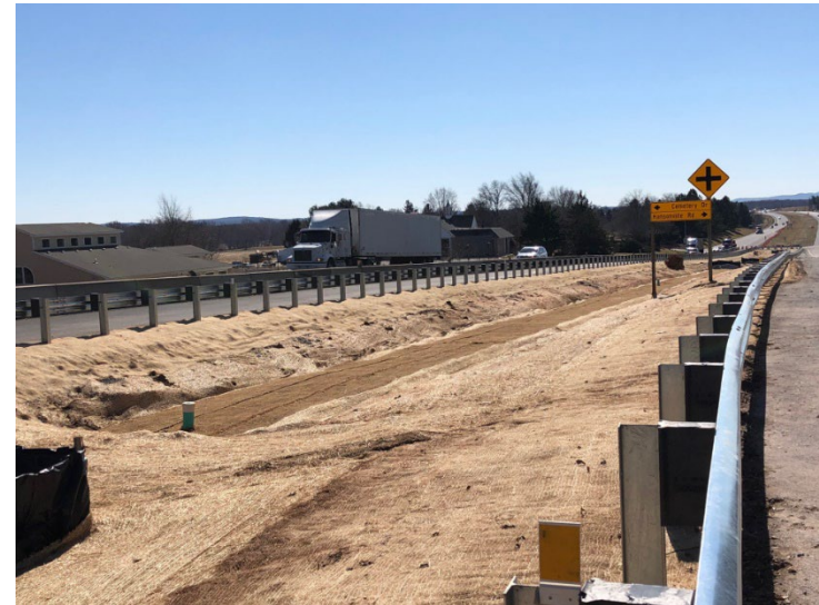
Bioswale under construction (US Rte. 15 near Frederick)
