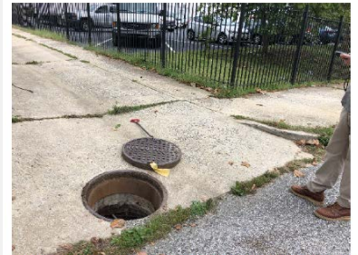
Figure 1: Storm sewer manhole & overflow outlet location
