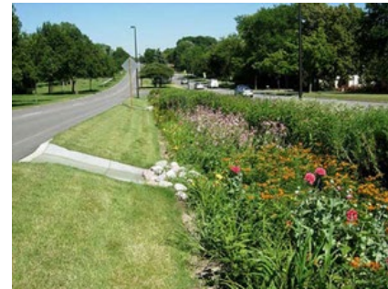
Below: Examples of roadside bioretention areas.
