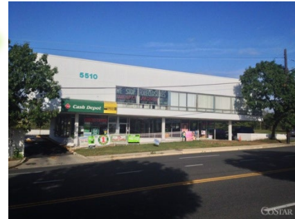
Above: Current Cherrywood Lane Conditions.
