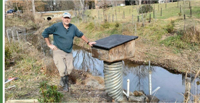
Keith Eshleman (UMCES) Plum Branch stormwater monitoring station (Ellicott City, Howard County, MD)
